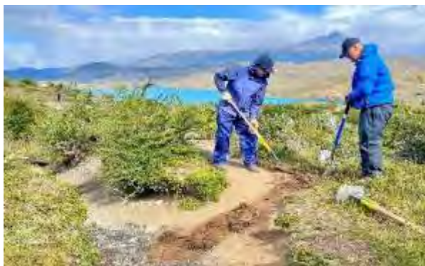
Figures 24-25 (Left-Right): Travelers begin construction of new water bars, cutting into established banks.
