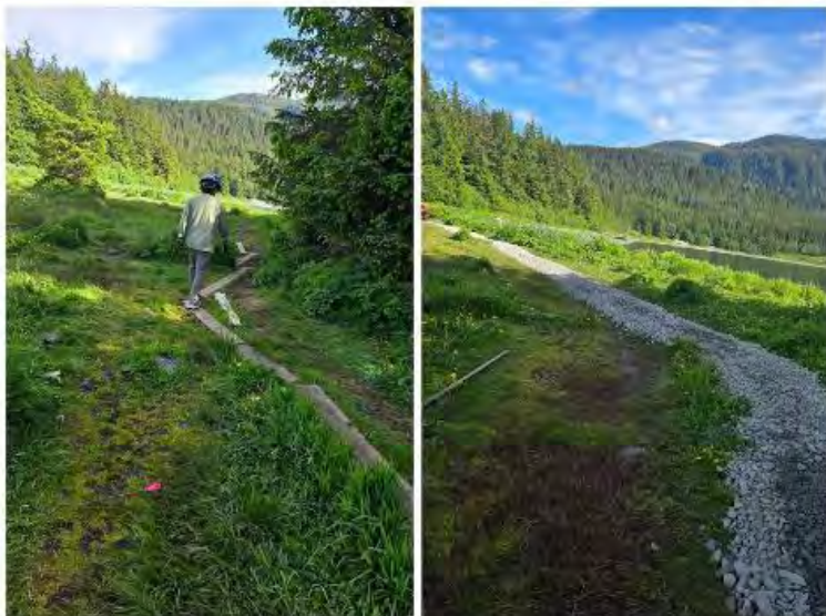
Before and After Photos of Point Louisa 400-foot trail foundation construction
