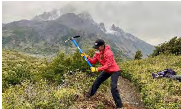
Figures 24-25 (Left-Right): Travelers begin construction of new water bars, cutting into established banks.
