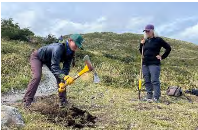
Figure 21: A team of 2 begins construction of a new water bar.
