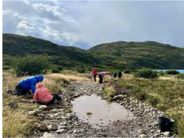
Figure 36 (Top Right): the group revegetates a puddle bypass and provides rock fill to allow the main trail to be passable.
