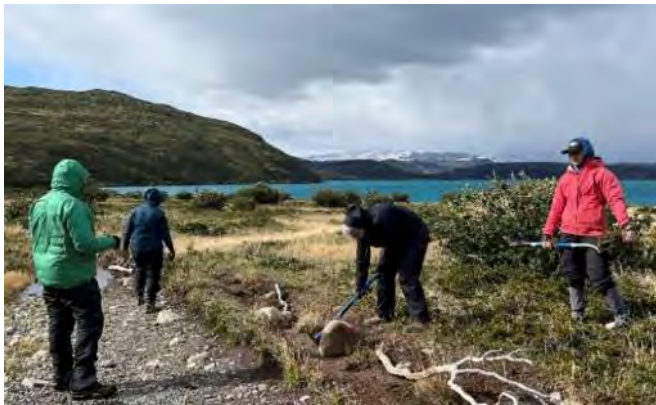
Figure 36 (Top Right): the group revegetates a puddle bypass and provides rock fill to allow the main trail to be passable.
