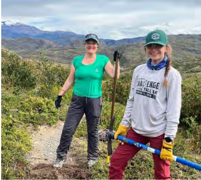
Figure 22: A team of 2 pauses construction of a new water bar
