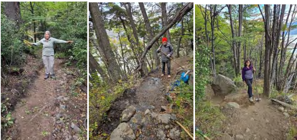
Much needed brushing, drainage repair and preventive drainage work
