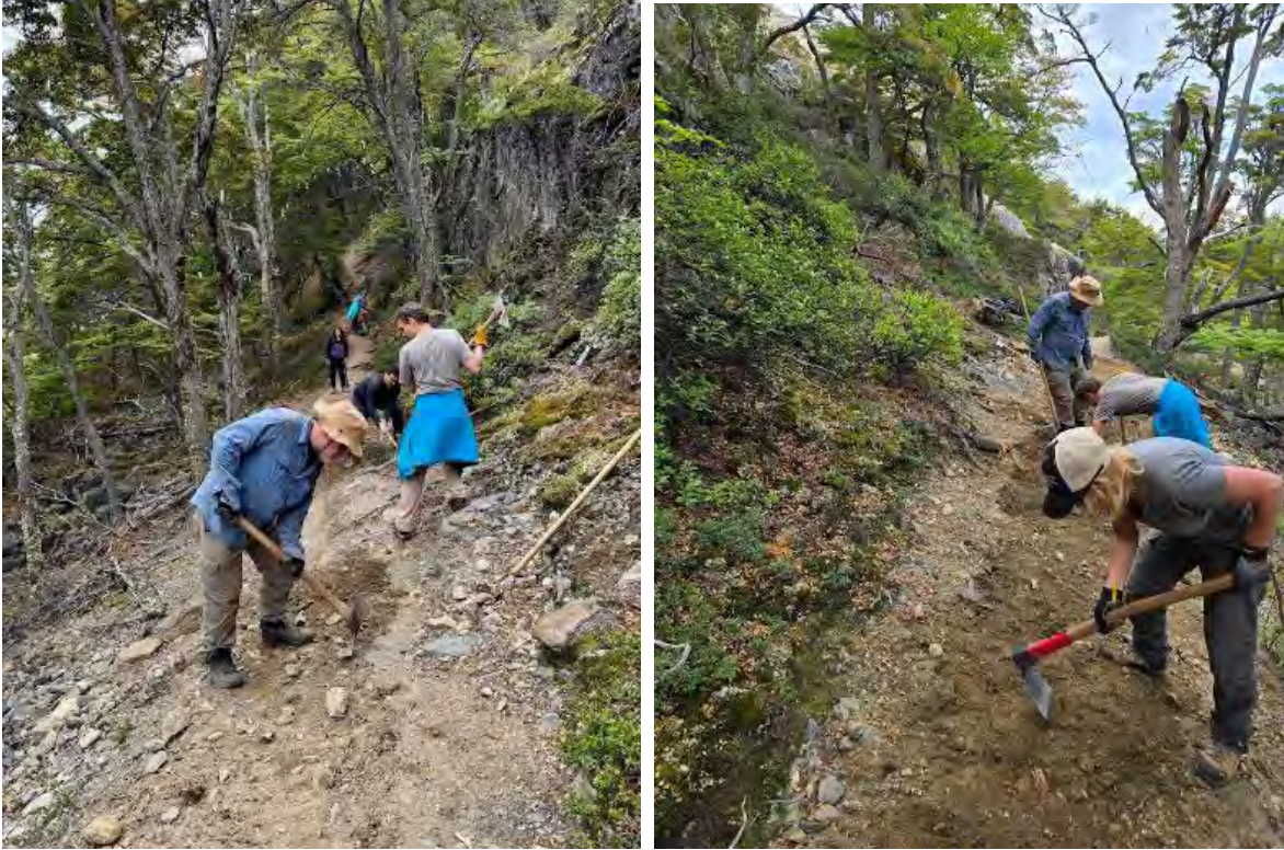
Trail alignment and leveling
