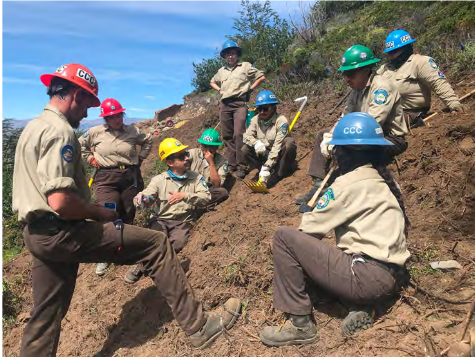
CCC crew discusses trail construction specifications.
