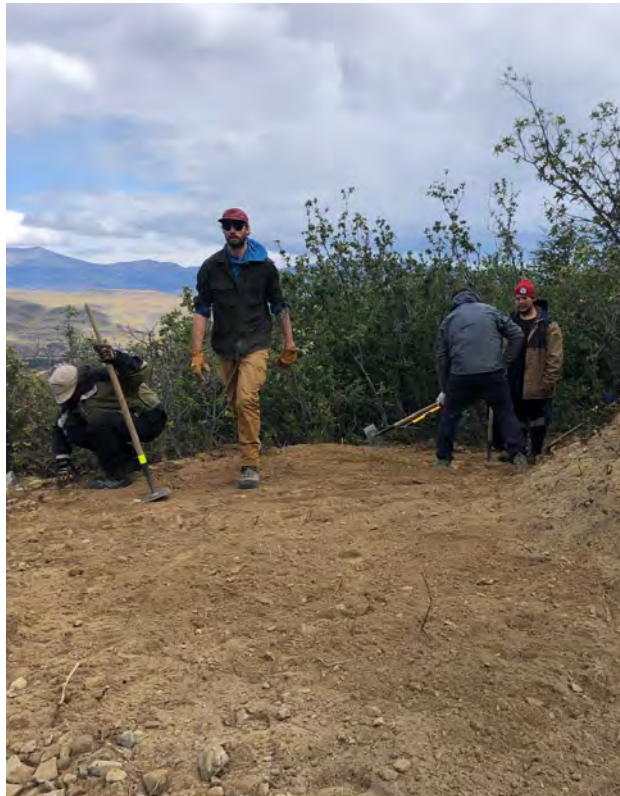
Fischer and AMA crew working around Rocky Point
