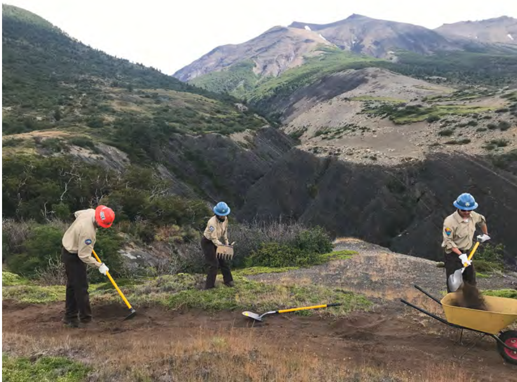
CCC crew working tread on new Base Torres Trail
