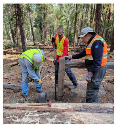
Part of the team took on the fencing project. The post and rail fence project included clearing debris from the ground, digging new post holes, and cutting and fitting rails to size. After the fence was tamped in and stabilized. leaf litter was returned to give the area an undisturbed appearance, and the roads and walkways were cleared of any leftover debris. At the end of the day the volunteers installed 16 new fence posts and 360 feet of fence.
