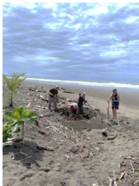
Two pits were dug and filled with fallen and sprouting coconuts and covered creating a small sea barrier.
