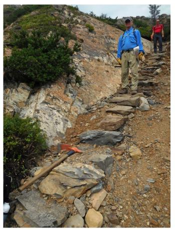
Fifty-five feet of rock walls were constructed to support the downhill side of the trail on steep slopes, 35 rock steps were installed in a very steep "chute", forming a very impressive rock ladder to make this section safe for hikers, and seven rock water bars were constructed to minimize erosion of the trail tread.
