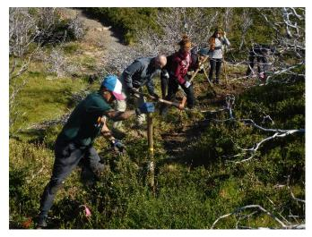
Working together, the group constructed about seven-tenths of a mile of new trail. Work consisted of determining the trail location, cutting small trees and brush - - with special care needed to cut the calafate bushes with their impressive thorns - - and removing vegetative material - - no small task as some sections of trail had brush with a deep root mass - - and removing soil and rock to rough-in the trail tread. After the brushing and roughing in of the trail
