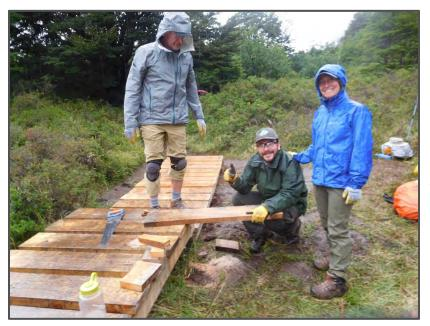
Much of the boardwalk was assembled using lag screws and battery powered drill-drivers, which was fast and provided an extremely strong structure. Because on-site CONAF rangers asked us to build more boardwalk than we had originally planned, the remainder of the boardwalk was built using nails.
