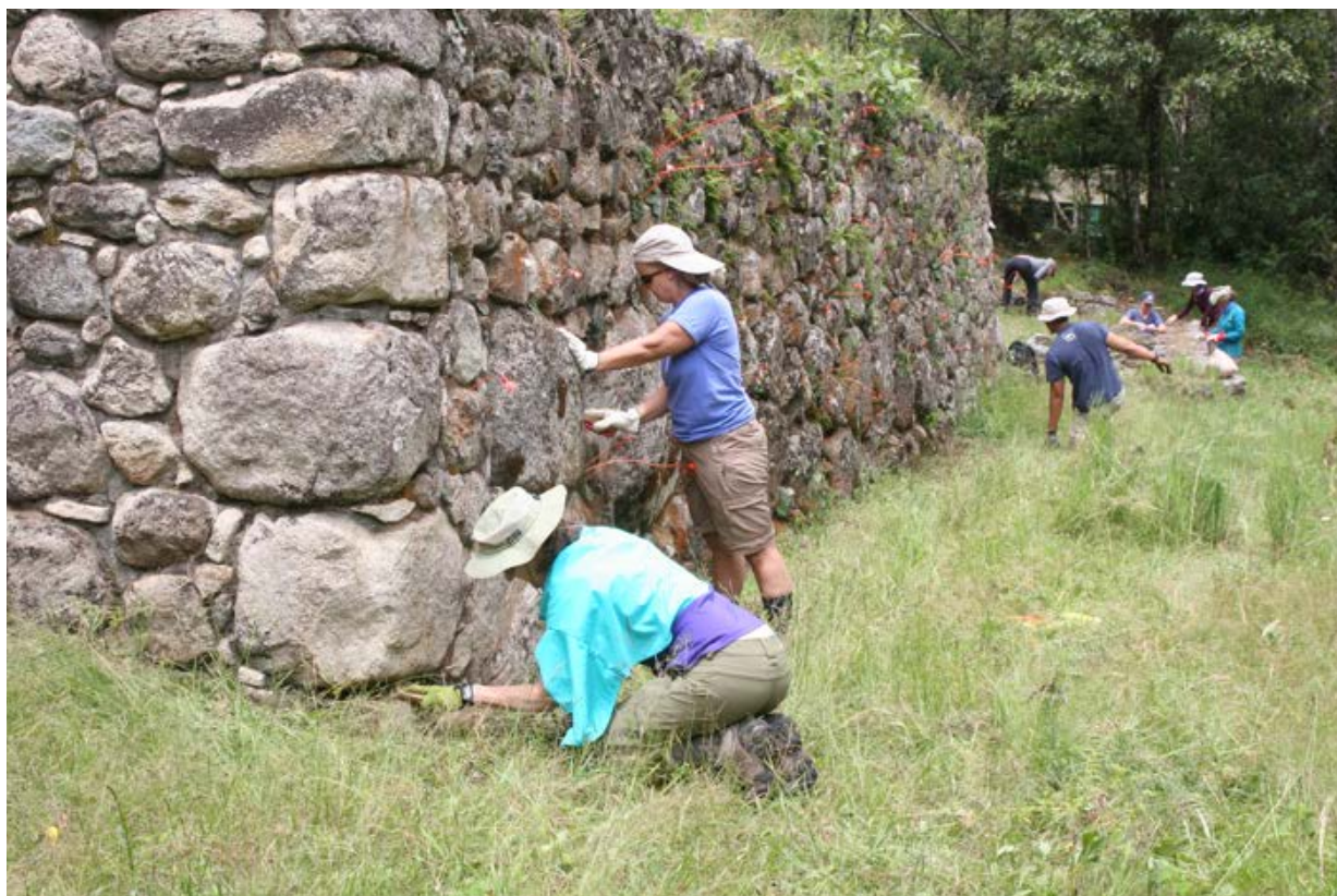
Figure 1 Volunteers cleaning walls and fountains at Chachabamba
