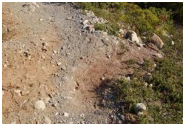
Example of Drain on Trail
