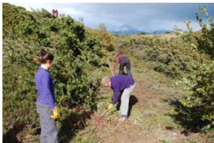
New Trail Construction, Clearing the Vegetation
