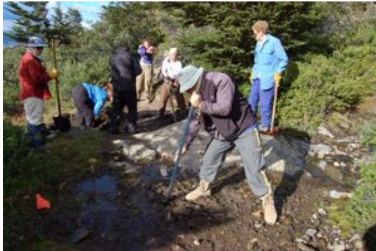
Removal of Rocks Near Stream Crossing
