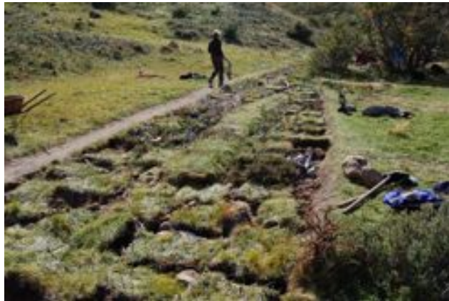
Grass and Shrubbery Plugs in Meadow Trail - Remaining Path was later Scarified for Seed Embedding
