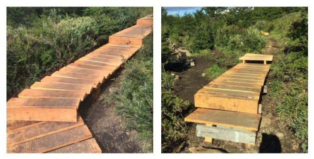
In addition, 90 feet of existing boardwalk was refurbished. Refurbishing the existing boardwalk consisted of rebuilding the decking utilizing used material scavenged from piles of discarded materials that were nearby. Finding good material took time, but in the end, a good boardwalk was assembled.
