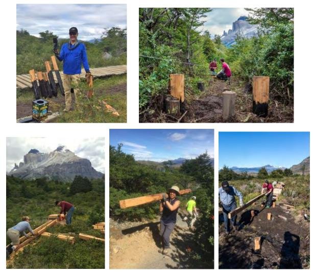
Initially, making the vertical posts was very time consuming, as it was a one-person job, cutting cypress logs into 3-4 foot pieces using a brushing saw, and then sharpening one end with an axe. On the third afternoon, CONAF delivered a chain saw for our use, and this greatly simplified and sped up the process. The stringers and decking required only occasional cutting to length.
