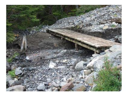
• We widened and improved (rock removal, raised profile, X-section correction) approx 60 yds of trail and added 6 rock steps, 4 water bars, and 2 side drains.
