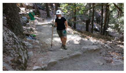
The third category was repairing and maintaining the designated mule trail between Happy Isles and the Vernal Falls footbridge. This was a difficult project that involved removing large rock pieces and using sledgehammers to break down larger rocks into smaller pieces that could be used in maintaining the trail. The volunteers also used rock bars to move and reposition large rocks to ensure a safe and stable trail for the mule teams.
