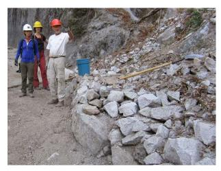
The first group set to repairing a section of trail where a boulder and several large rocks had shifted into the trail. Their primary goal was to reconstruct a 25-foot section of retaining wall and to shift the large rocks and boulder off the trail. This group also repaired an additional section of retaining wall roughly 3 feet long.
