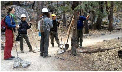
toward the lake clearing and constructing approximately five drainage areas to aid in removing water from the trail.
