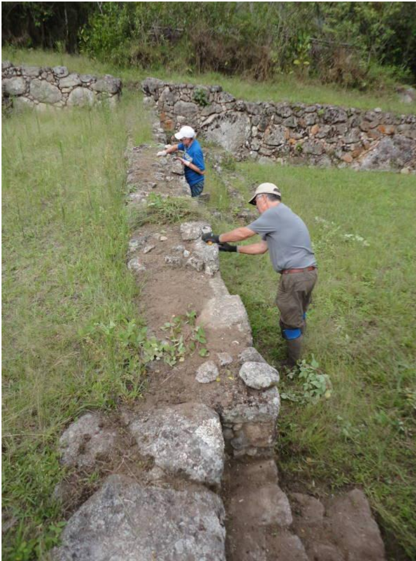
Removal of plant material from terrace and water fountain at Chachabamba.
