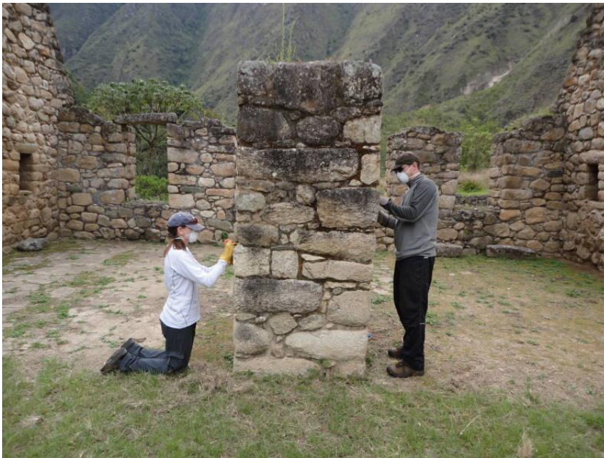
Volunteers carefully removing plant and moss from stone pillar. Chachabamba.
