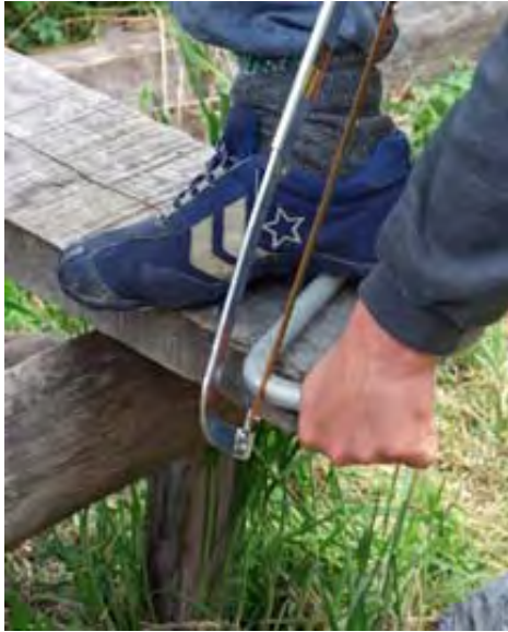
Bolts were hand cut and filed
