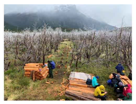
Then the layout of all the posts were marked on the ground and the installation of the cypress posts began. We needed two posts on seven-foot centers installed into the ground for 560 feet. Each hole needed to be dug and posts carried to the site and pounded into place.
