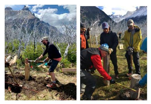
Once the posts were secured and leveled, a beam was attached to the post and leveled to hold the stringers.
