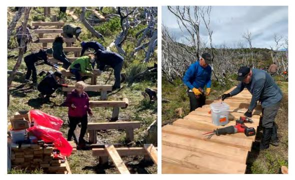
We also needed to build a bridge across a live stream. The bridge was built with two eighteen-foot stringers and we applied the appropriate decking. Secured to the boardwalk, this provided a safe and effective crossing of the stream.
