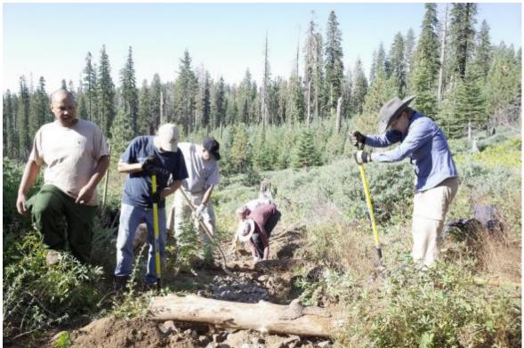
Inserting logs to prevent rutting of the trail.
