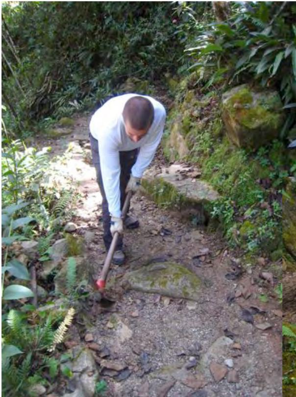
The entire length of the Putucusi Trail from the trailhead to the landslide (approximately two miles) received maintenance from volunteers. In addition, 19 water drain structures, such as the one below, were added to protect the trail from erosion.
